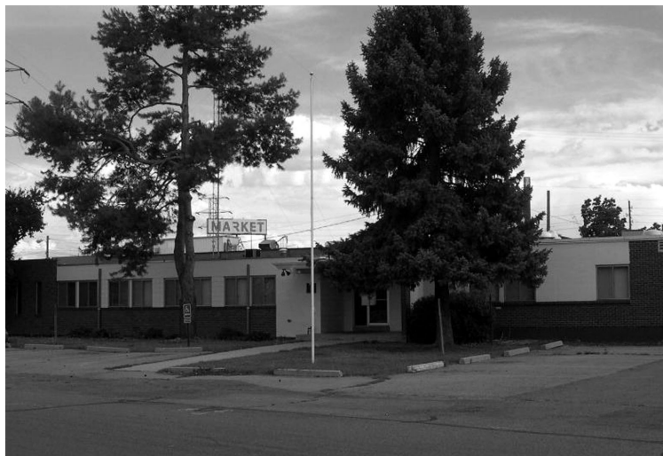
New SRM headquarter's building.
