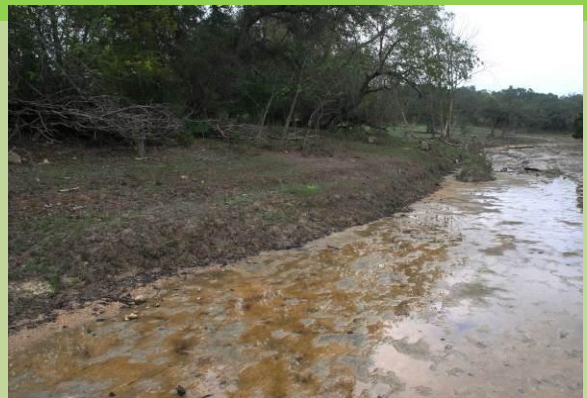
A riparian area “losing ground”: With inadequate vegetation to dissipate energy during high flow events, channel, banks, and floodplain are subject to excessive erosion.
